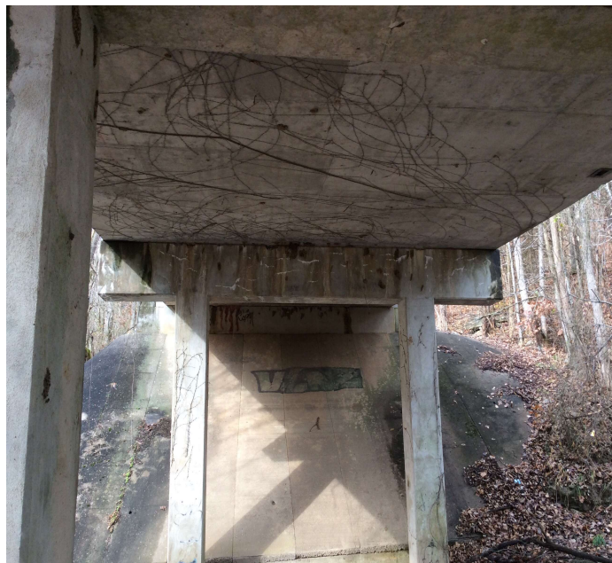
PHOTO 1 Description Bent # 3 Span # 2 cracking with efflorescence.
