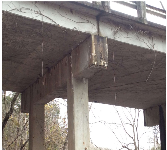
PHOTO 2 Description Bent # 3 left edge of the cap cracking with efflorescence.
