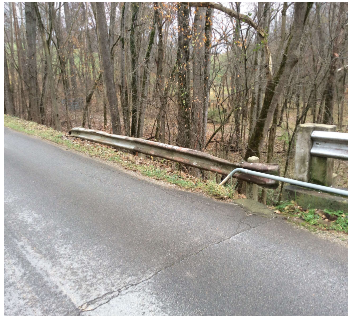
PHOTO 2 Description South west approach rail damage.
