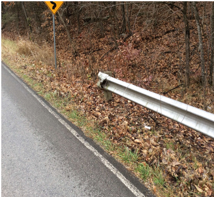
PHOTO 1 Description North east approach rail damage.
