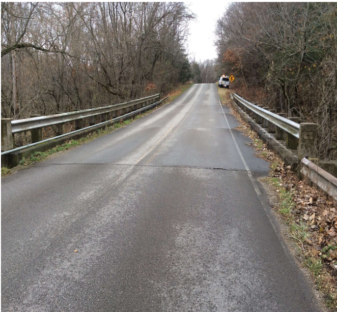
PHOTO 1 Description Vegetation and debris in the deck gutters.
