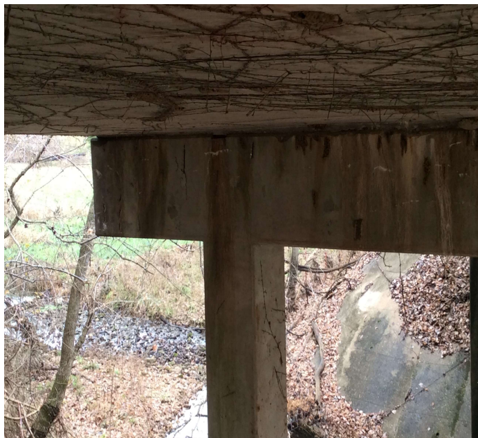
PHOTO 3 Description Bent # 3 Span # 3 vertical spalls with exposed reinforcing steel.
